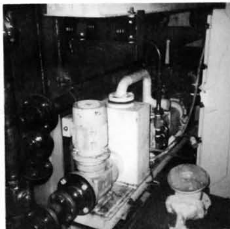
The vacuum-pump raft for Terra Nova's blackwater system.
