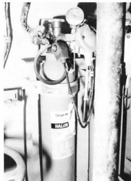
Fire protection at what environmental cost? The DDH-280 and FFH-330 classes rely heavily on halon 1301 systems such as this one on board HMCS Halifax .
