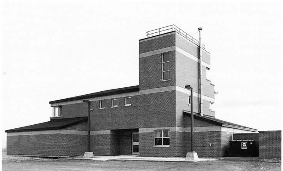
The William MacKay Creelman building at the Fergusons Cove Influence Range
