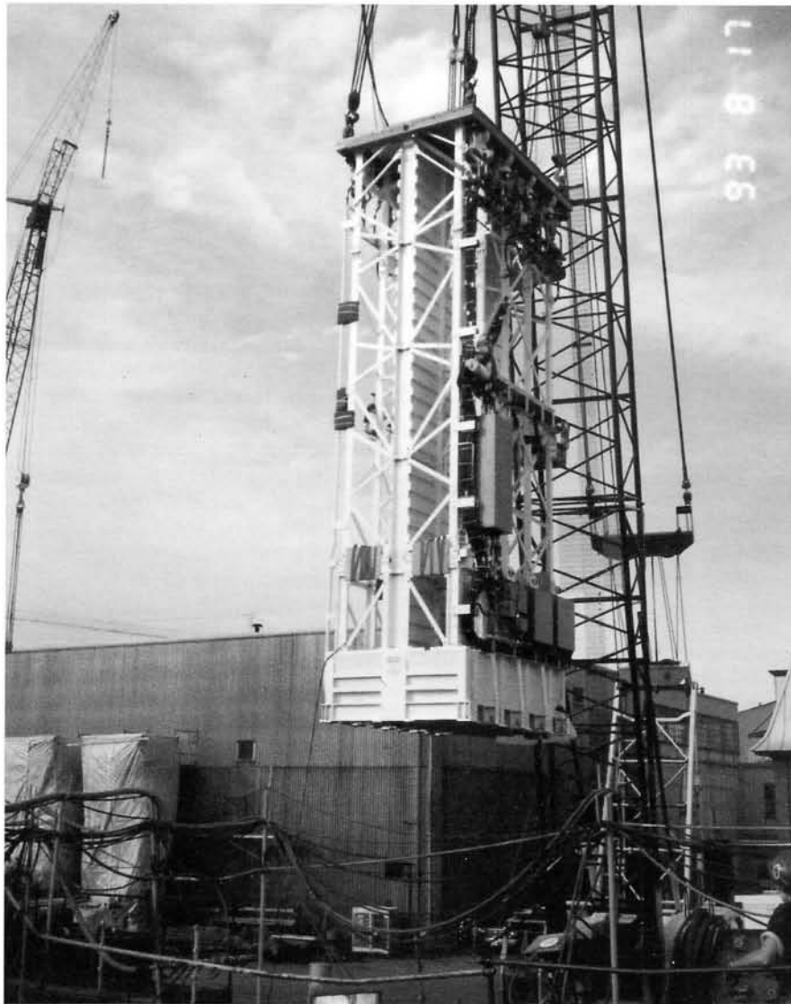
Fig. 7. A module is transported to the ship by crane during module load-out.
