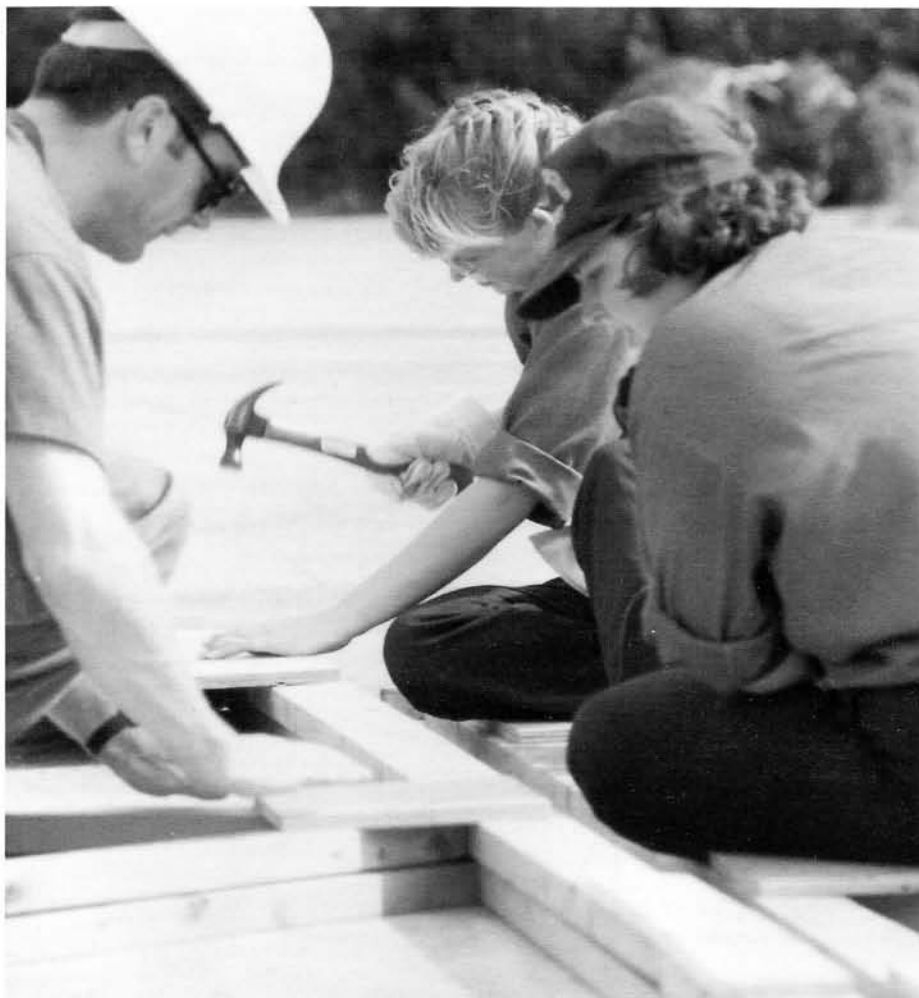
Capt. MacGougan of the CFB Halifax Base Construction Engineering section works alongside LSET Burke and Pte (Storesman) Pye.
