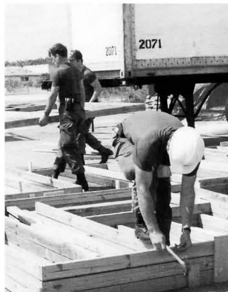
Canadian crews prefabricate frames and trusses for the 1992 Hurricane Andrew relief effort in the Bahamas.
