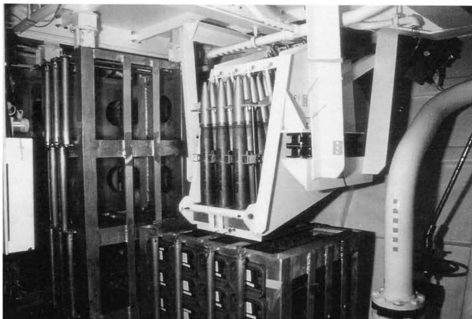
Some of the instrumentation details are visible in this view of the 57-mm ready use racks. Note the static-g gauges to the right of the inert shells. These simple “drop and tell” gauges are easy to use, but rather limited in detail. Note also the aluminum housings for the piezo-resistive accelerometers fitted above the light-coloured fixture on the left of the photo. (NETE photo by George Csukly)
