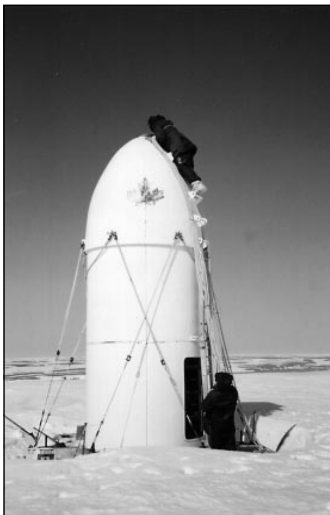
Attaching the lifting bridle to a silo.
