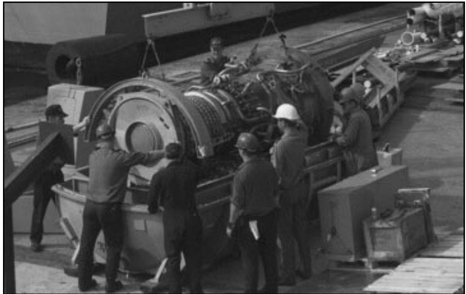
The new gas generator is hoisted out of its shipping "coffin."
