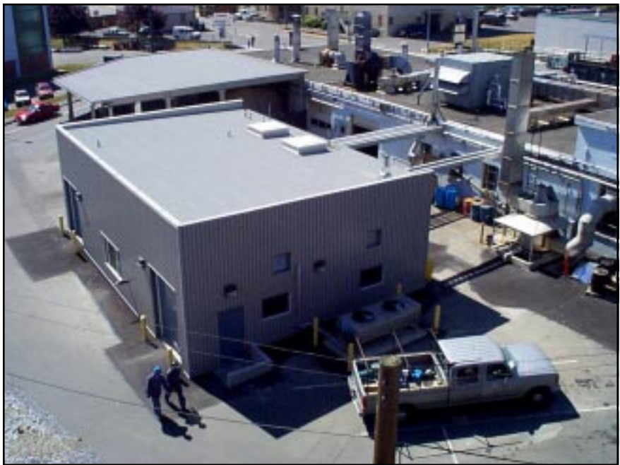
Fig. 1. The waste treatment facility at FMF Cape Breton's dockyard electroplating shop. (DND photo.)
