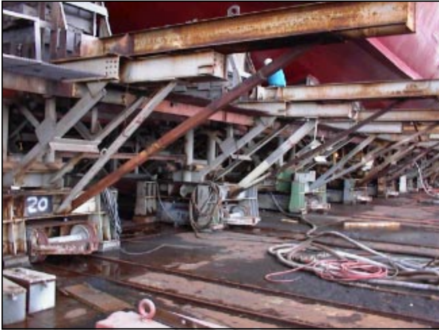
The ship construction cradle for the USS McFaul rests on a series of electric trolleys that will eventually transport the fully assembled DDG into the floating drydock for launch and final outfitting (see photo on previous page). (Photo courtesy Ingalls Shipbuilding)
