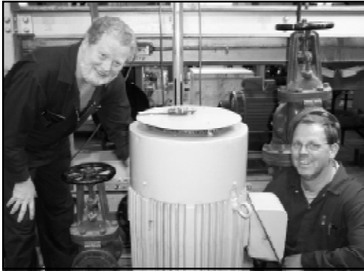
Veteran fitters Duncan MacGregor and Robert Leslie carried on with a pump installation even as the minister's tour passed through.
