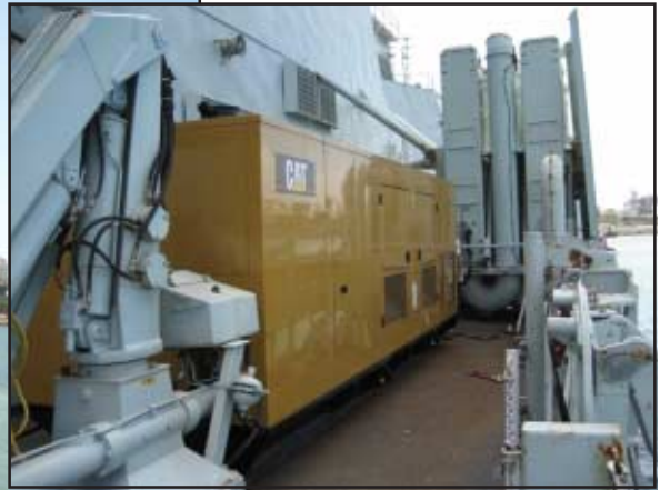
A tight fit on the port side. A less-than-ideal sling mechanism and minimal clearances on the superstructure complicated the installation.
