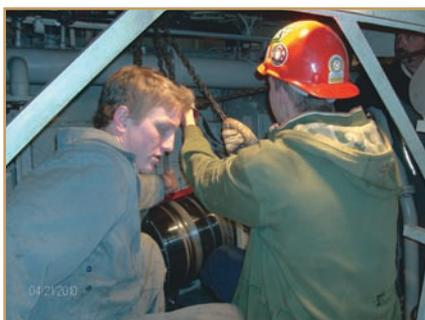
Step 8. FMFCS mechanical apprentice Jake VanRossum (left) and FMFCS rigger Justin Burke rig the new 265-kg clutch in place.
