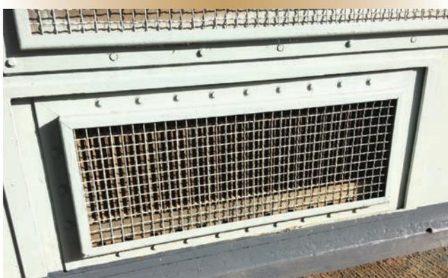
Figure 2. A manually operated air intake bypass louvre.
