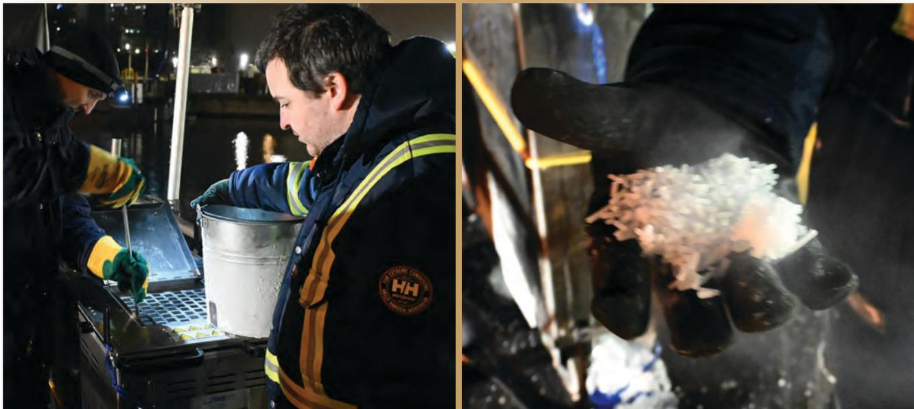
Technicians from the FMFCS Submarine Electrical shop prepare the dry-ice pellets (right) in the open air, jetty-side.
