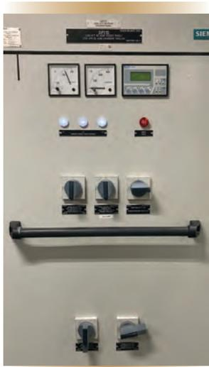
Figure 2. Main 220-V aft de-icing feeder panel.
