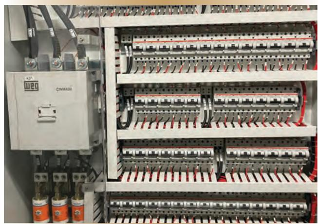
Figure 3. De-icing heating panel showing breakers.
