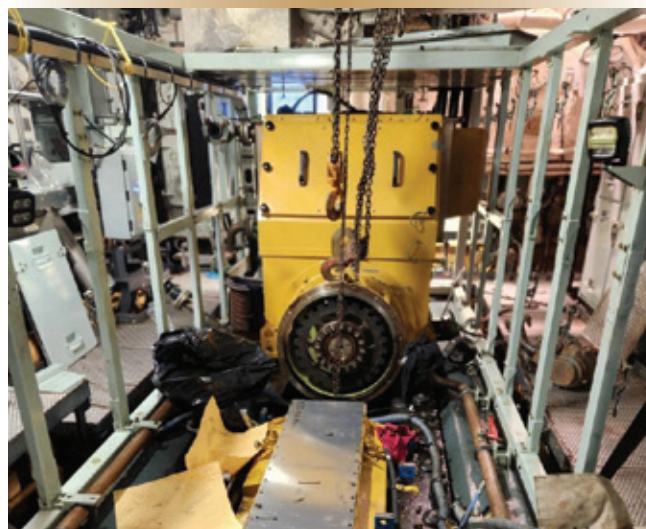
Enclosure disassembled, generator moved, damaged engine removed
