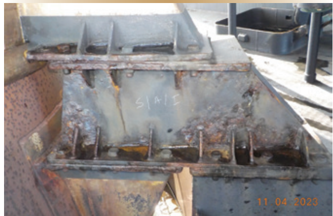
Corrosion – Seatings/Brackets
