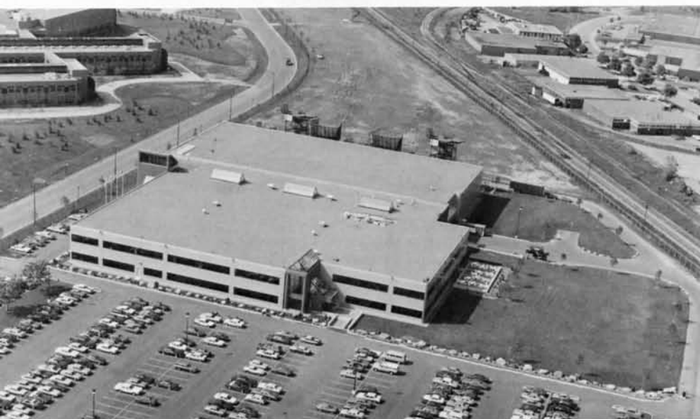
Paramax's Combat System Test and Support Facility in Montreal's Cité Scientifique. Note the radar test field in the background.
