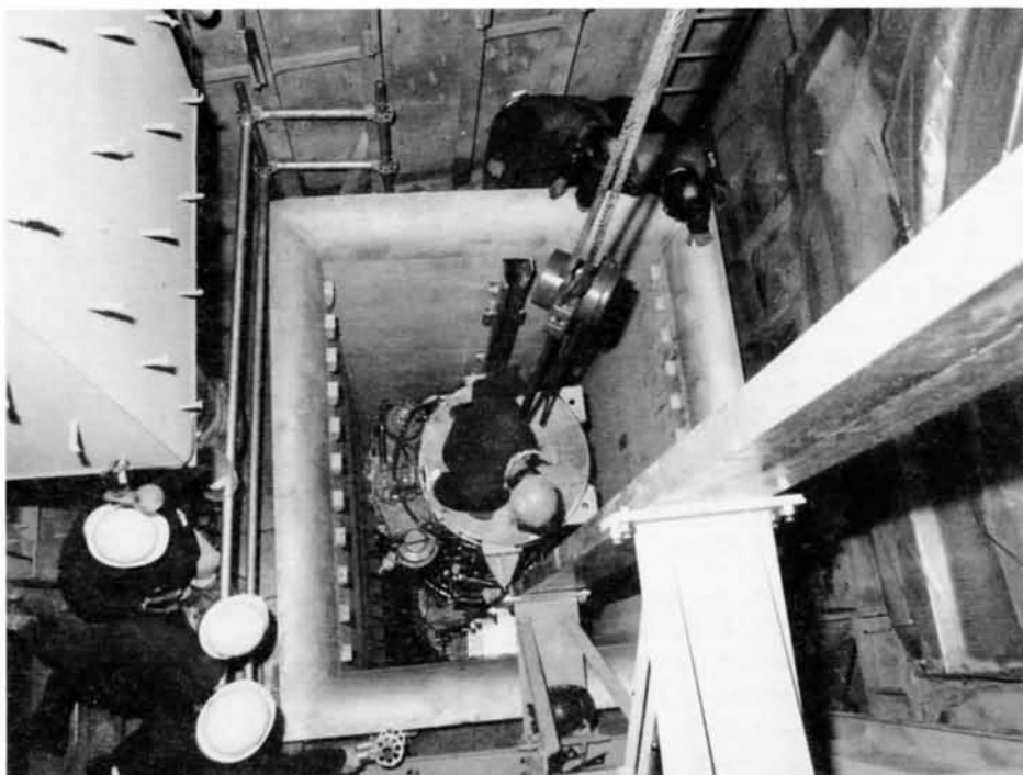
Fig. 5 An overhead view of the gas generator on the chain hoist as it clears the critical region.
