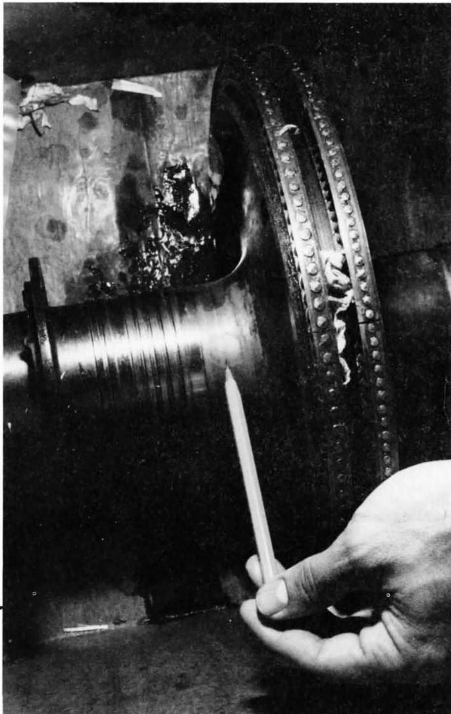
Fig. 4. An acid etching process was used to reveal this hot spot.
