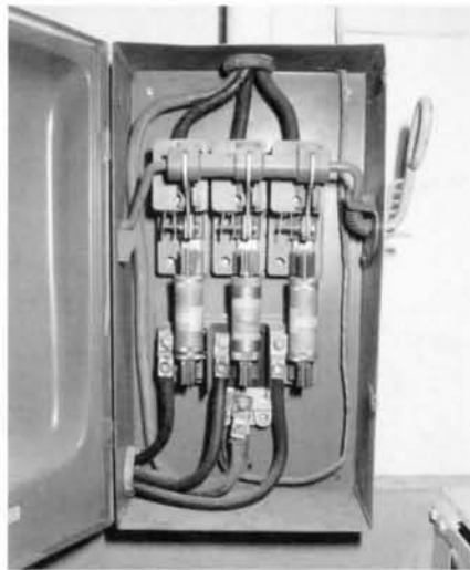
The components of this fused disconnect switch appear normal in visible light. However, in the IR thermal image, the whiteness of the cable, fuse and switch on the left reveal an abnormally hot area indicative of a problem in the electrical circuit.
