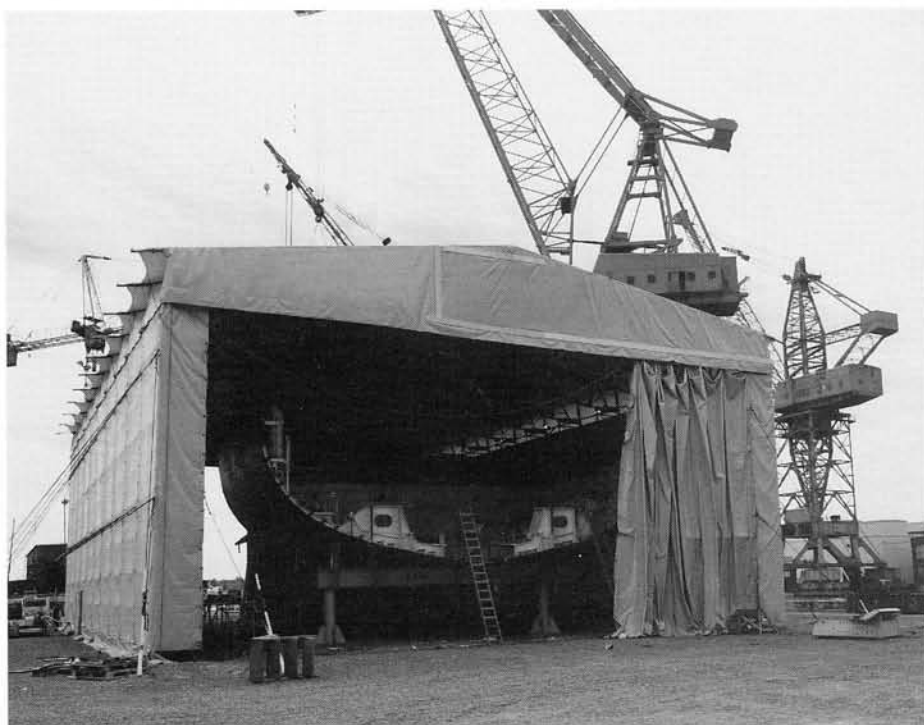
Fig. 8. HMCS Halifax Temporary Shelter
