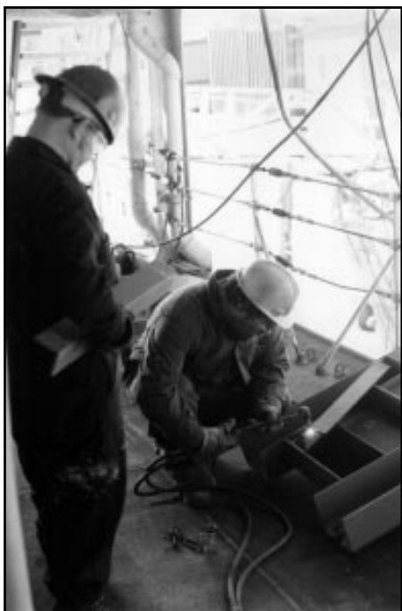
Preparing seatings for the torpedo handling system.
