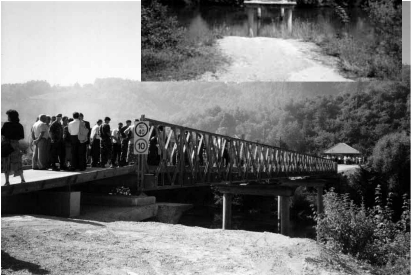
The destroyed bridge at Blatna (inset) was rebuilt as a combined Canadian-British project to allow Serbs to return to Avanska. For two weeks while the nearby Otaka bridge was being rebuilt, this single-lane track was a major route to Croatia.
