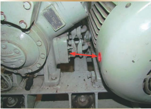
Figure 2. Close-up view of the limited space between the motor and compressor. The oil sight glass is to the left.
