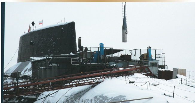
De-fuelling the Russian nuclear-powered submarines involved lifting the radioactive spent nuclear fuel assemblies out of the reactors in transfer flasks, then containerizing them for safe shipment to a processing facility in the Ural Mountains.
