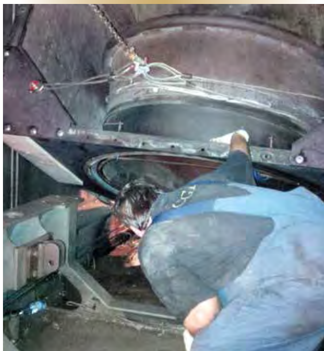
Figure 8 – FMFCS rigger Steve Eddy guides the exhaust duct into a horizontal position.
