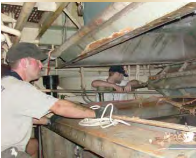
Figure 6 – With the exhaust expansion joint moved forward, FMFCS rigger Spartius Toope (left) and plater Ryan Shaw have cleared the way for the exhaust duct to be rotated into position for removal.
