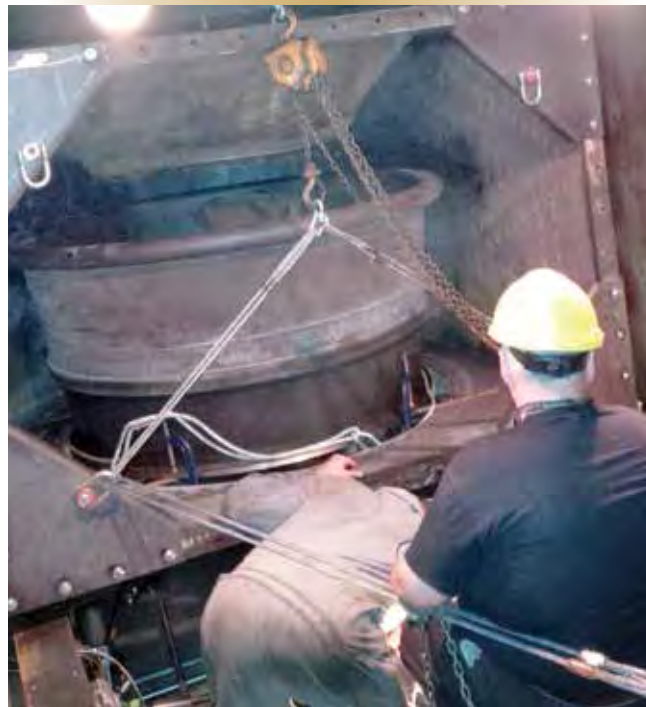
Figure 9 – Clearances were as little as 3 mm as the exhaust duct was moved carefully through the enclosure for removal.
