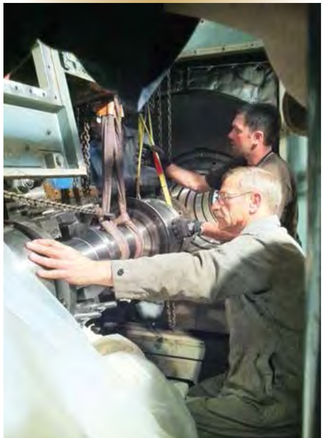
Figure 11 – Things begin to come together. With the new exhaust duct in position, the author (foreground) and FMFCS rigger Spartius Toope can install the replacement GT input shaft.
