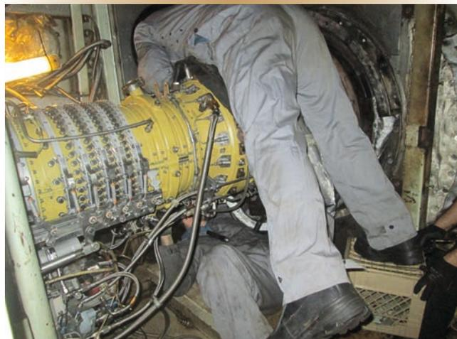
Figure 9. Allison Gas Turbines FSR Russ Brown ensured the alignment between the engine output and the gearbox was absolutely straight.
