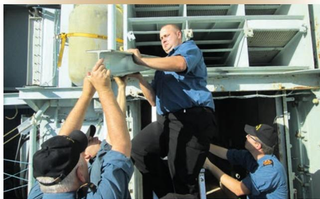
Figure 2. Installing the lifting beam.
