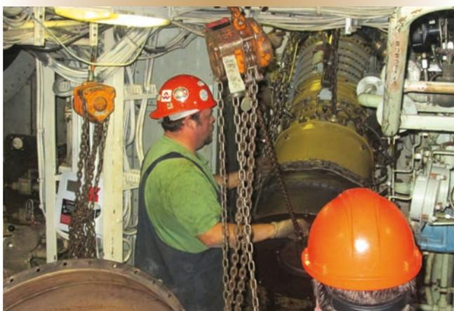
Figure 8. The new engine is eased carefully into the enclosure.
