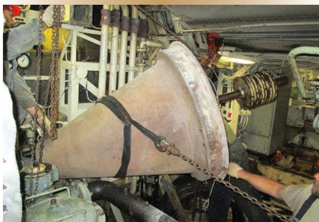
Figure 4. Removing the diffuser cone.
