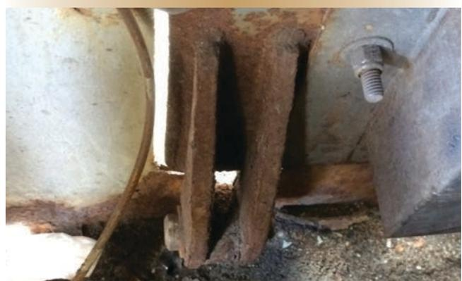
Figure 3. A bypass louvre hinge and hinge pin seized through corrosion.
