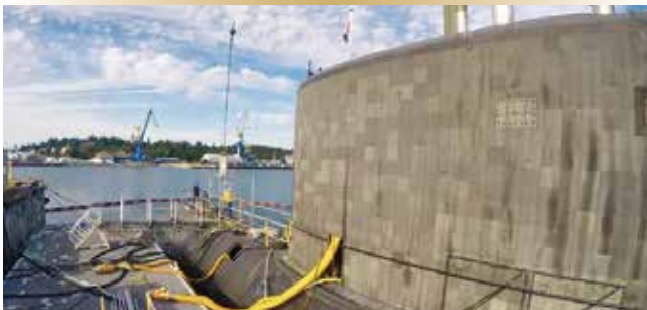
All 480 battery cells had to be removed from each submarine before the replacements from Victoria could be installed on board Chicoutimi .
