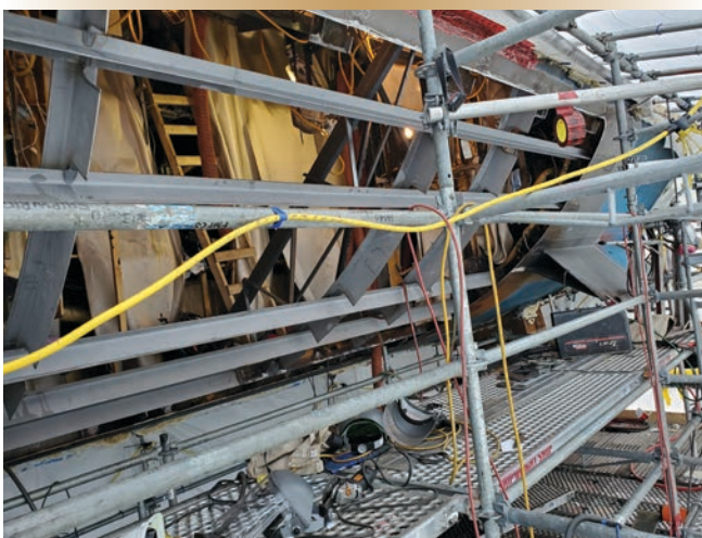
Figure 1. Scaffolding set up inside the weather enclosure, with the ship's side plating and section of angled bilge keel removed.
