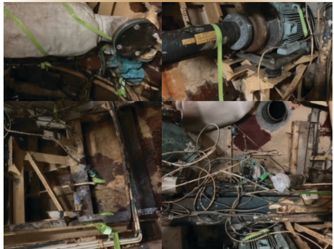
Figures 2a & 2b. The first hurdle was to finish removing the many interference items inside the ship that were blocking full access to the frames, longitudinals and hull plating.
